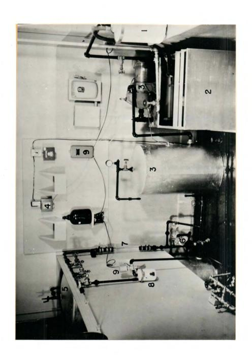
Figure 5. Flow-through diagram of superchlorination-dechlorination pilot plant
